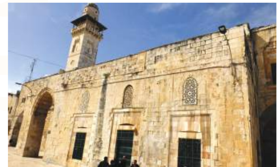
Exterior of Madrasa al-Ashrafiyya (MT Archive)
