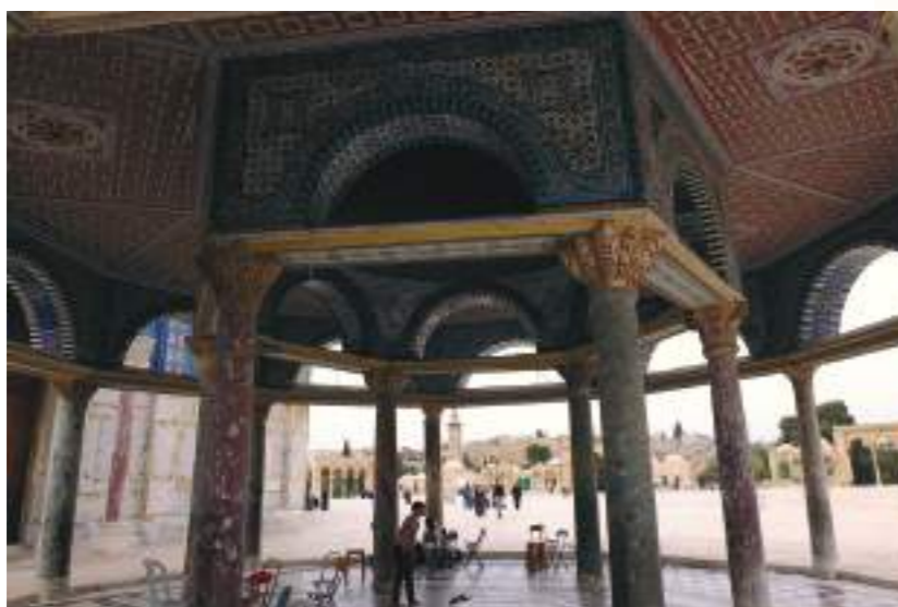
Image 25a. Inside view of the Dome of the Chain (MT Archive)
