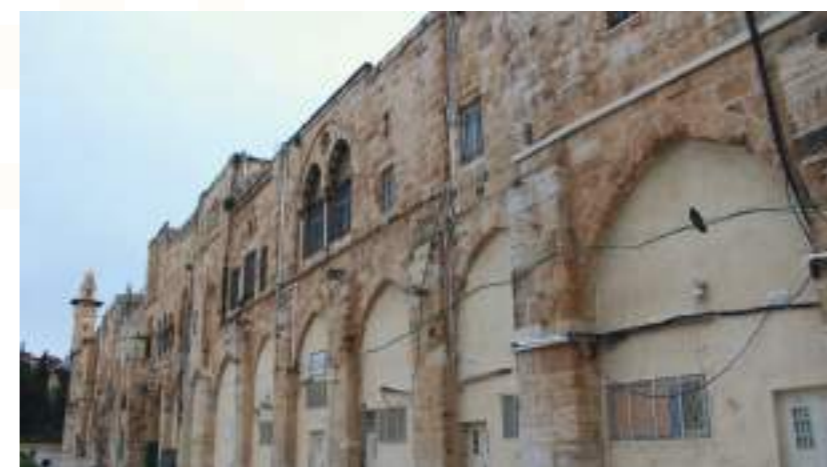
Image 55.14-55.15. The northeastern and northwestern cloisters of al-Aqsa Mosque and Madrasas al-Dawadariya, al-Basitiyye, al-Aminiyya, al-Farisiyye, al-Is'ardiyya, al-Melekiye, and al-Javiliyye above them from east to west (IYV Archive)
