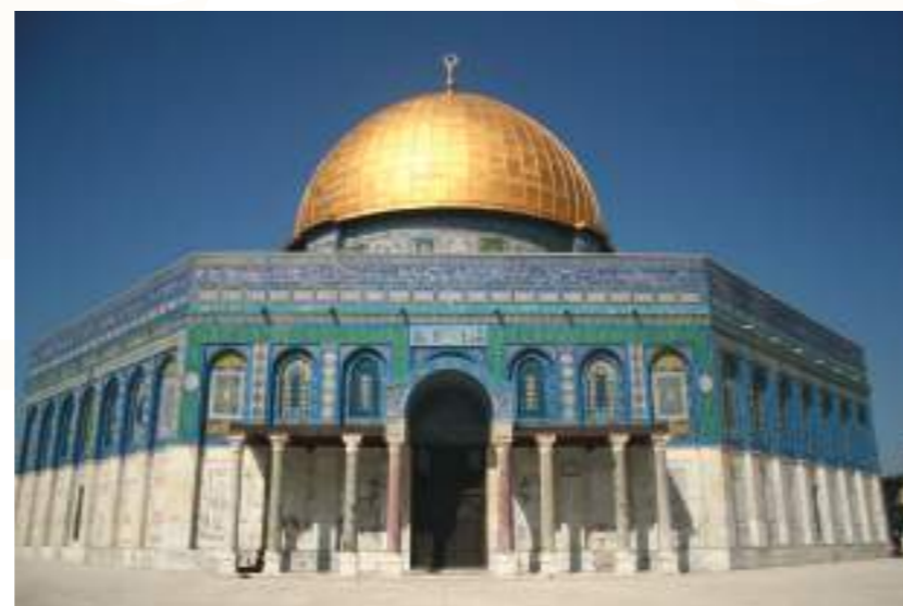
Image 27. The view of the door entrances to the Dome of the Rock that in later years were superimposed on the columns by opening up the marble porches (FA Archive)
