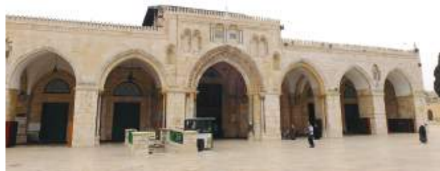
Qibly Mosque's North Facade Stonework
