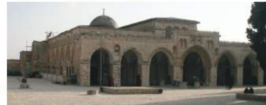
Image 11. The seven-pointed arches of al-Masjid al-Aqsa (remaining from the 12th-century Crusaders) with its front (north) entrance and the entrance to the basement, which was used as a synagogue by some Jews and a small mosque by Muslims (FA archive).
