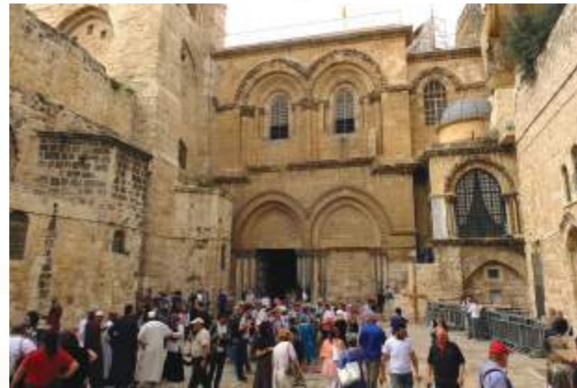
Image 21. Aerial view of the double-door entrance and courtyard of the Holy Sepulcher Church 25
