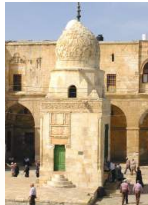
Sabil Qaitbay of al-Aqsa Mosque
