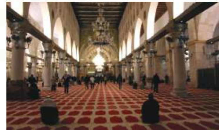
Image 12. The wider middle nave of al-Aqsa Mosque. A general view of the wooden-clad beams that were rebuilt after the 1969 fire between the staged columns (IYV archive).
